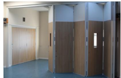
Two folding wall partitions have been installed, using part of a legacy from Bruno (Peter Burton), a former GSL. They were part of the original plan of the building and make a very flexible set of spaces. The Main Deck can be split, with a smaller River-end space, or the Ward Room can be expanded to include this space.
